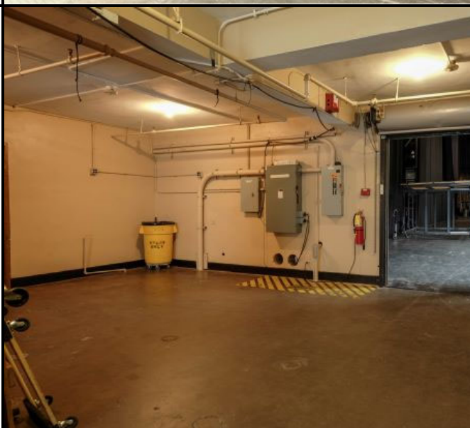
STAGE LEFT- OFF STAGE PROP ROOM
