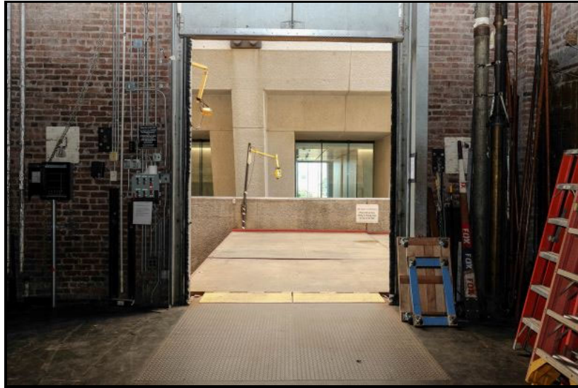
LOADING DOCK DOOR / DOCKS VIEW FROM STAGE
