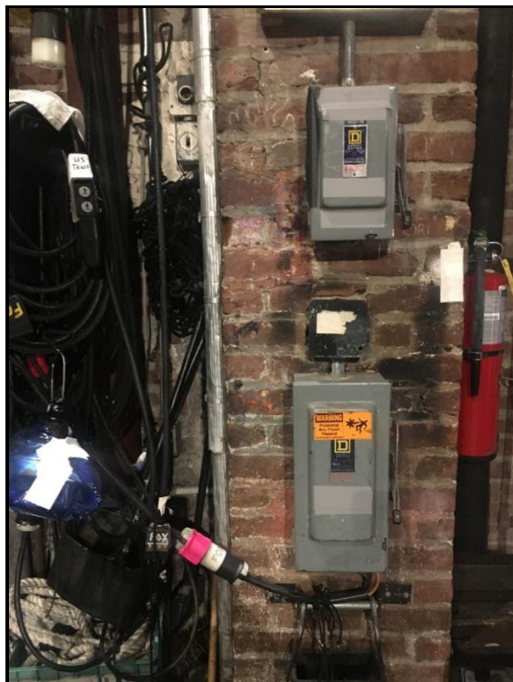
POWER DISCONNECT UP STAGE RIGHT (USR)
